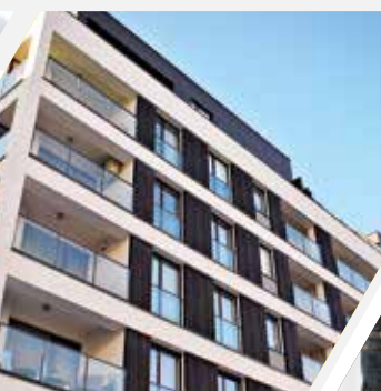
Portonovi 2017 - 2019 Novi - Montenegro Residential buildings
